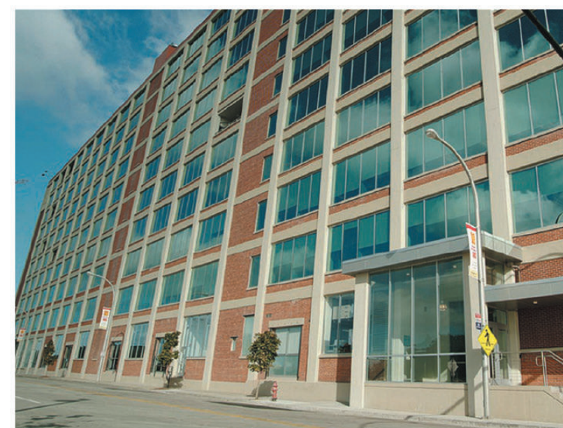
LCO Building in New York 23XRV500
