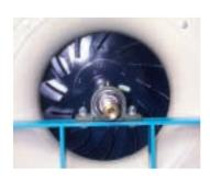
Forward Curved impeller constructed from galvanised steel sheets is designed to meet high volume, medium static pressure and low-speed operation. Backward curved impeller is made from solid steel with enamel paint finish. Typical application is in medium to high static pressure, non-overloading and high-speed operation. Other fan type of different characteristics may be custom selected and built to meet specific
