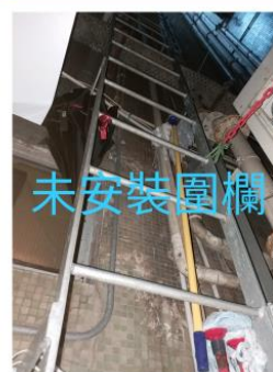
Fixed Ladder Inspection Job Site: Eva Court
